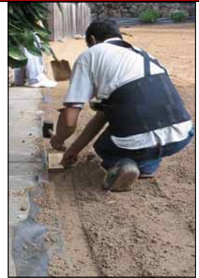
Hand tamp hard edges using a spare piece of 2 x 4 wood and rubber mallet. This helps to set final level and insure a clean edge.
