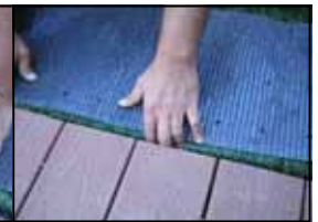
Check cut and fit and remove waste
