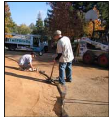
Hand tamp hard edges using a spare piece of 2 x 4 wood and rubber mallet. This helps to set final level and insure a clean edge.
