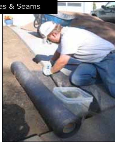
Hard edges should be cleared of all debris. Aggressive weeds and grasses may need additional treatment prior to laying base materials.
